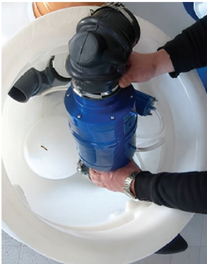
Faster installation and removal of the valve unit
